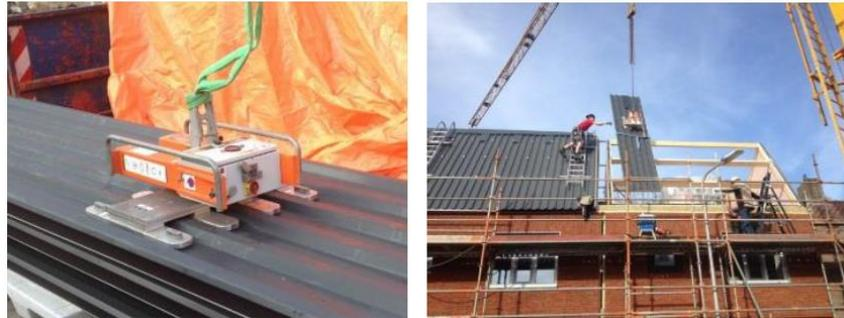
Figure 3: Roofing sheets were lifted piece by piece (Berben, 2015).
